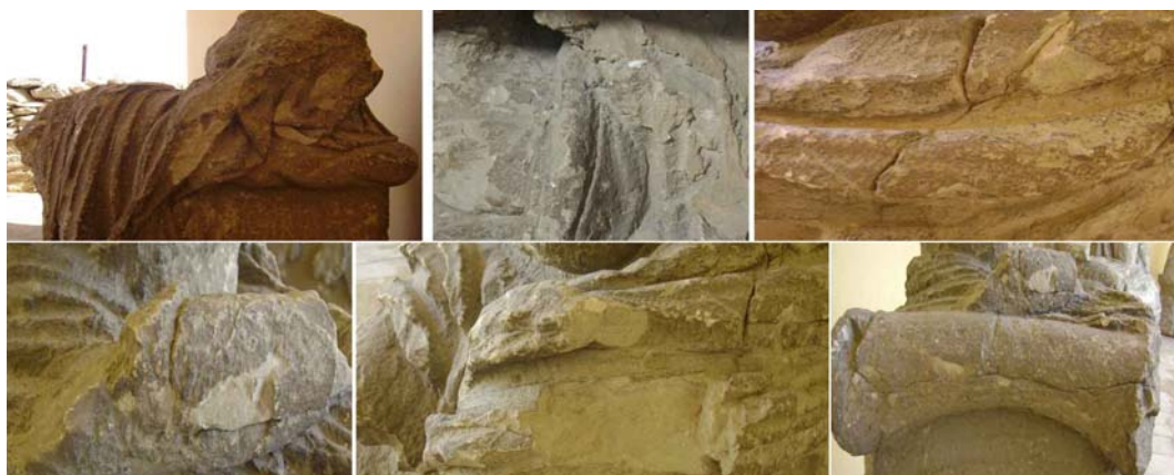
Fig. (2) Details of deterioration phenomena of the statues as surfaces degradation, crystallization of soluble salts, dark layers on the surfaces, vertical and horizontal deep cracks, erosion by wind effect and missing parts.
