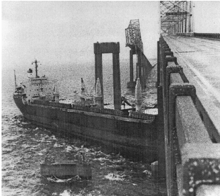
Fig. 1. The 1980 collapse of the Sunshine Skyway Bridge
