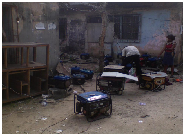
Figure 1: Cluster of Generating Sets
