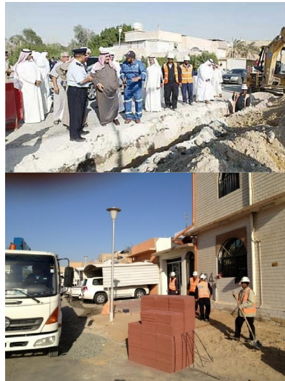
Figure 3. Sides of Gas-leakage treatment processes of at Block No. 1 of Al-Ahmadi Town.
