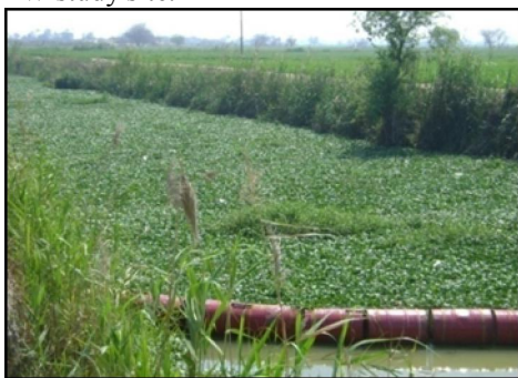
Plate (1): A free water surface wetland treatment system
