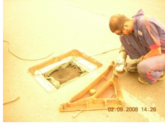
Picture (9) Adopting the manhole cover to the unit
