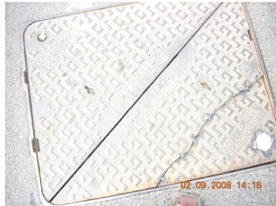
Picture (10) The cover of the MH after finishing the installation
