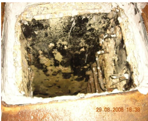
Picture (1) corroded MH sides and cover due to the emitted H 2 S
