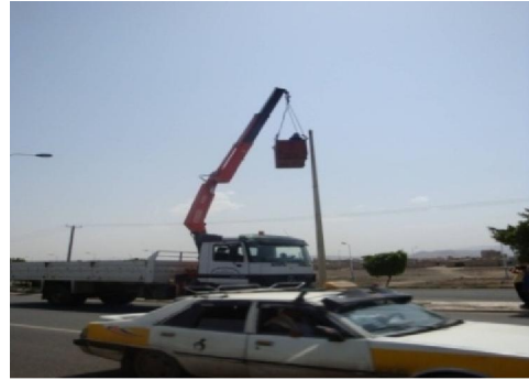
Picture (3) odor measurements at the ventilation column
