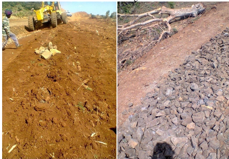
Figure 6: Human pressure on plant & soil conservation via infrastructure expansion.
