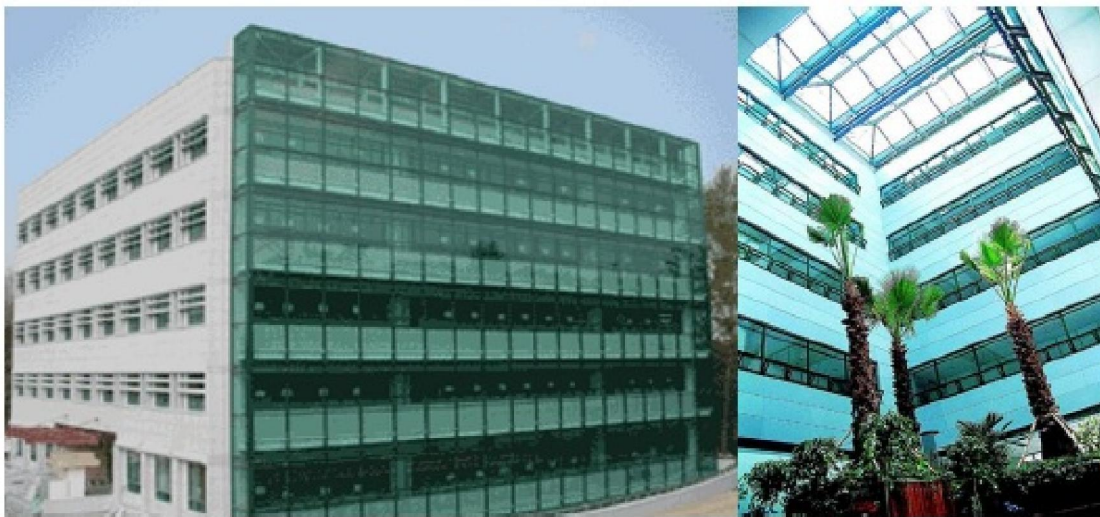
Fig. 2. Exterior and interior of Green building
