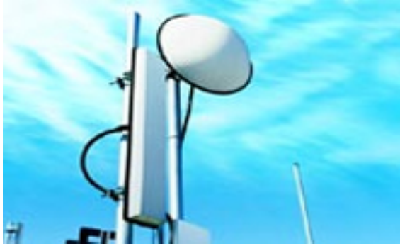
Figure1.2 WiMAX transmitting tower
