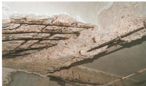
Fig.2. Shows the steel rust which leads to the fall of the concrete cover and cement on the column and ceiling[4].
