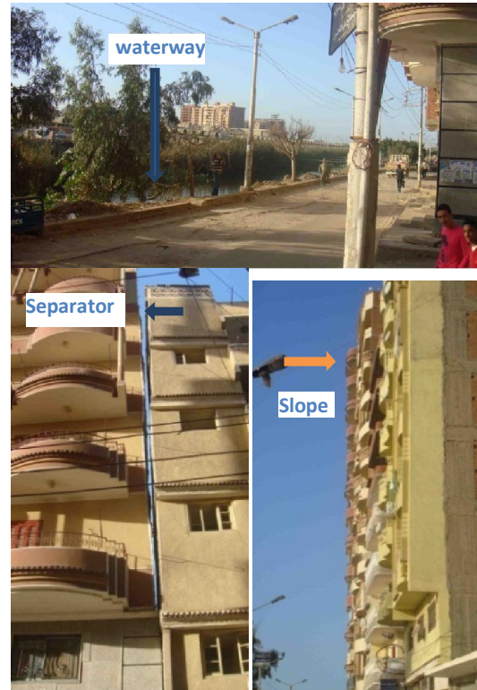
Fig.8. Gap between the oblique building and the adjacent neighbor [Author].
