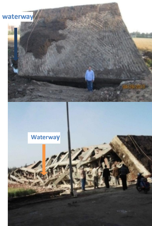
Fig.5. shows the collapsing of the building as result of the slide of its foundations` in the neighboring agricultural land [26,author].
