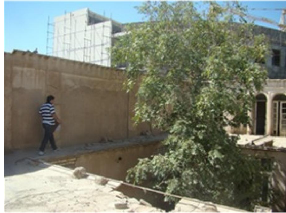
Figure 5: the outer courtyard of the civil house
