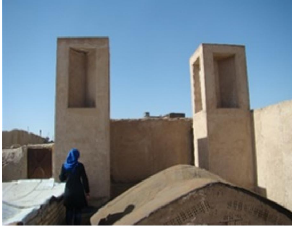
Figure 3: Wind catcher on the south side of Madani House
