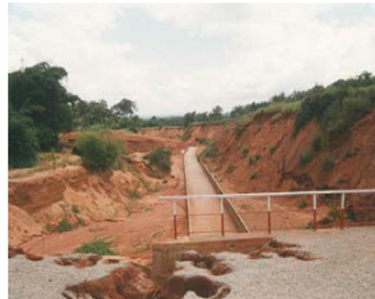
Figure 3. Gully erosion site in Amaokwe, Figure 4. A Gully site in Umuchiana, Aguata, Anambra State, Abia State.
