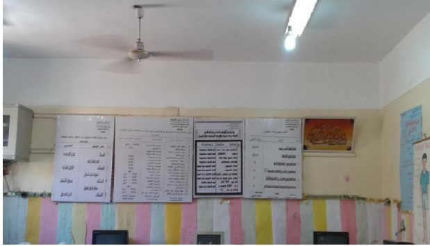
Picture NO. (3-5) the roof fan in classrooms, from researcher
