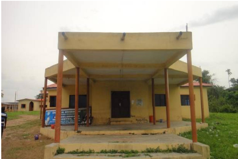
Figure 1: Grasses growing on the crack floors
