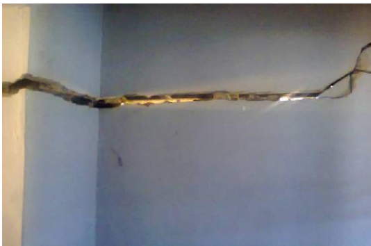
Figure 2: Sign of differential settlement
