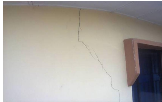
Figure 4: Cracks on the outside wall
