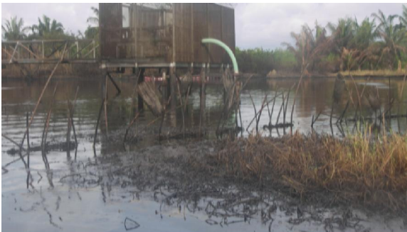
Plate 4: Chevron equipment failure spill site
