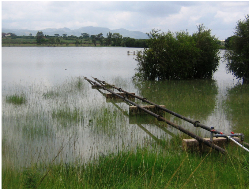
Plate 1. Water extraction pipes that supply water to a water treatment unit located nearby the reservoir.
