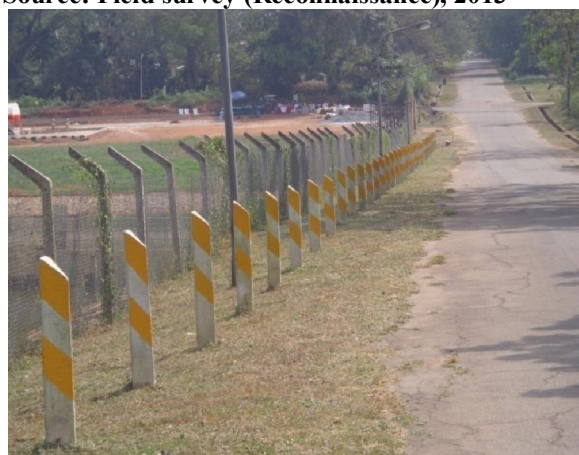
Plate 4.8: A section of the dam with a constructed road
