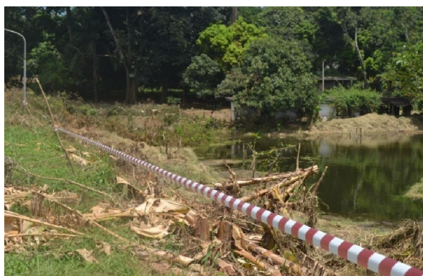
Plate 11: Awba dam during the reconstruction work Source: Field survey (Reconnaissance), 2013
