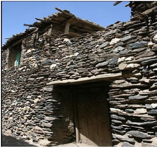
Fig. 2. Varkane's mixed manner of construction-stone ground floor and adobe for floors above.
